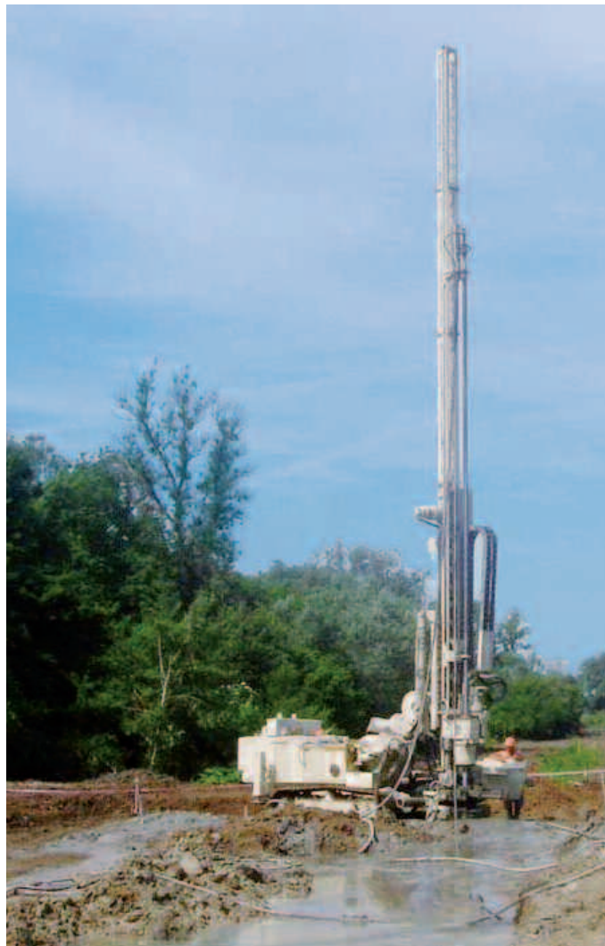
TWS1400-RAPTOR in cantiere, equipaggiata con traliccio jetting L = 12000 mm (lunghezza totale Mast: 18580 mm) TWS1400-RAPTOR on jet-grouting job site, equipped with jetting trestle L = 12000 mm (Mast total length: 18580 mm)
